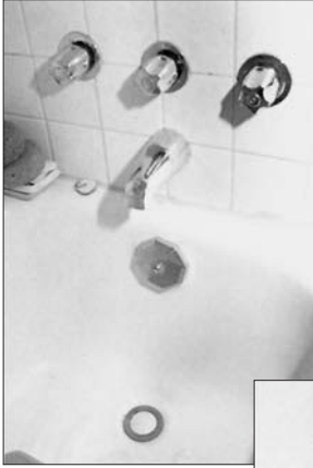
Taking a bath is safer and easier with a foot-activated drain plug.
