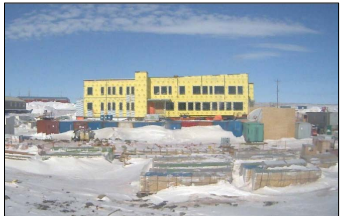
Construction of new Baker Lake head office.
